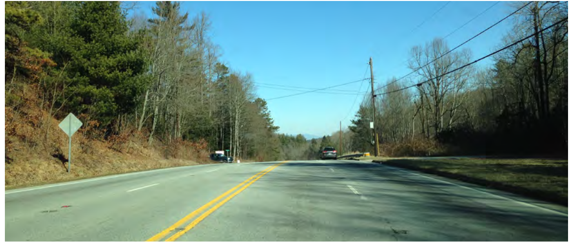
Existing roadway crossing section approaching Brevard, North Carolina.
