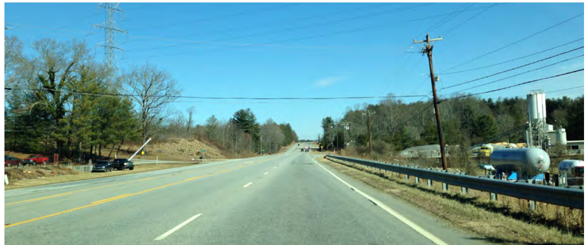
Existing roadway crossing section approaching Mills River, North Carolina.
