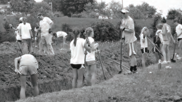
Below: Student volunteers dig lines for septic systems
